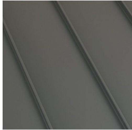
Metal Panel - Standing Seam
