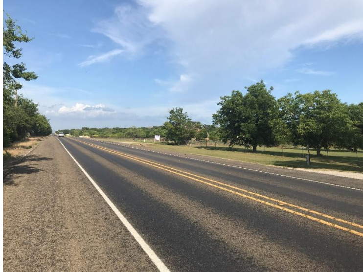
Drive 2 Looking East
