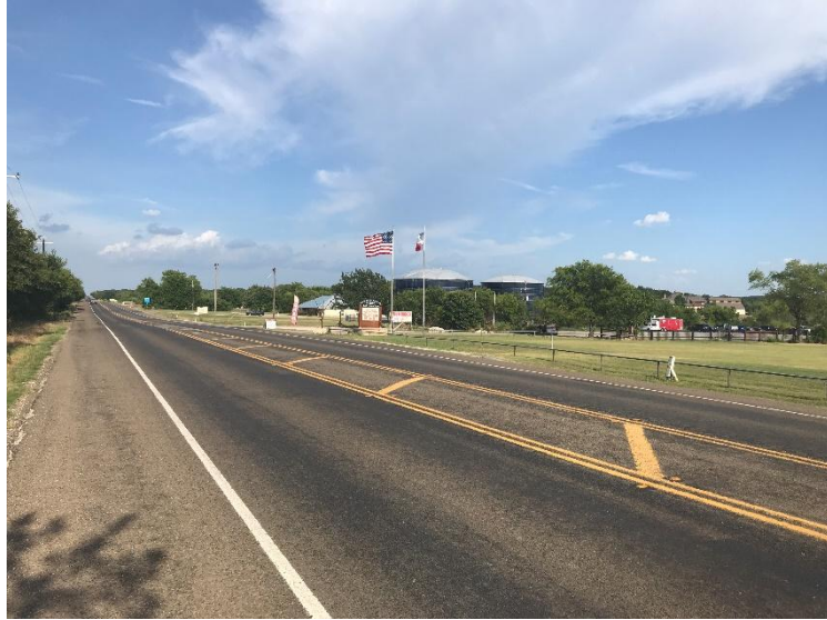
Drive 1 Looking East
